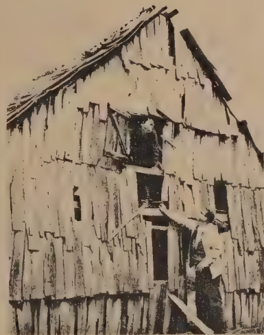
"EASY, CHARLEY!" — Charles Grace examines the loft of another style barn while Jim Coomes takes a safer look from ground level. Each Hensley Settlement family used its own style of architecture. This building originally had a double wall for insulation purposes.
